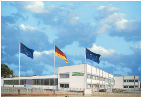
Production plant in Neuenhaus
