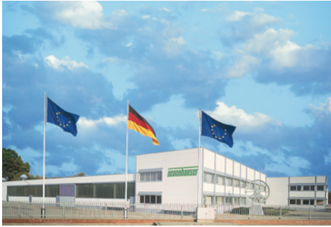
Production plant in Neuenhaus
